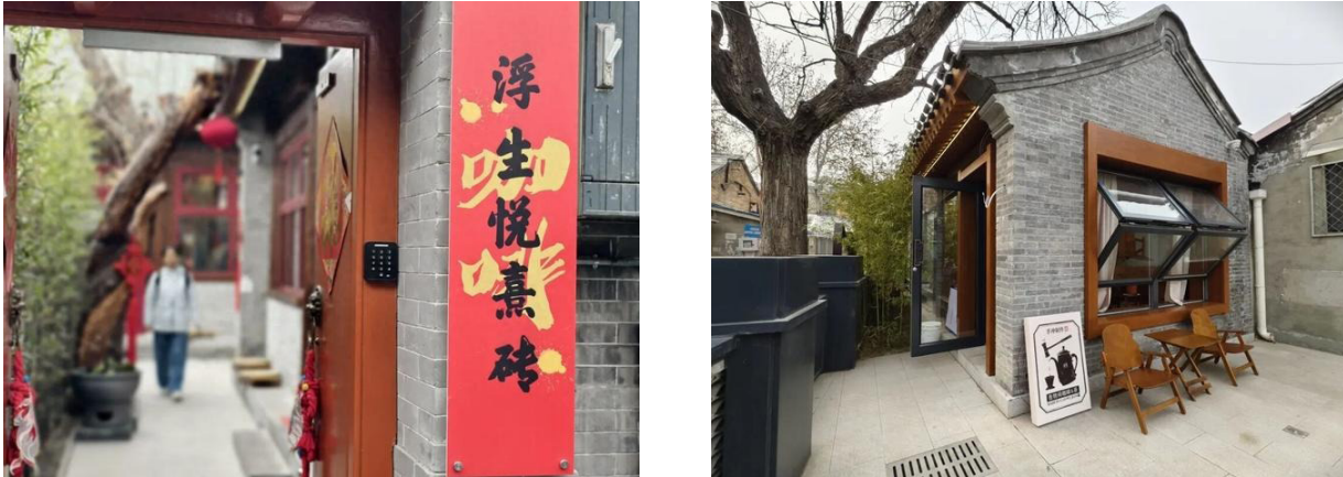
Figure 3. Contemporary photographs of the Caishikou West Area: (a) an offset entrance sequence in Xizhuan Hutong; (b) a repaired courtyard building with a clearly visible paved edge and drainage grille. Source: Beijing Xicheng Official Release (2026). Reference photographs, not taken by the author.
